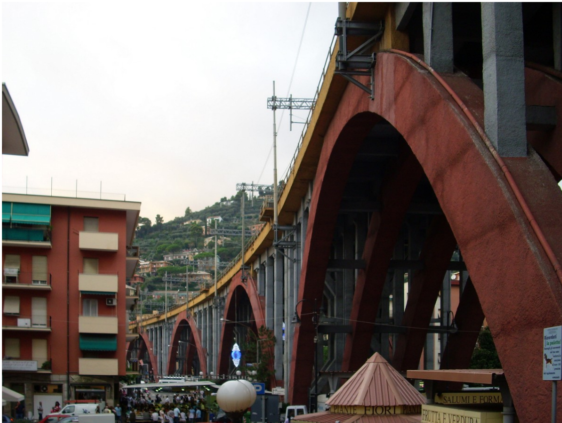
The railway bridge that crosses Recco in Liguria Italy
